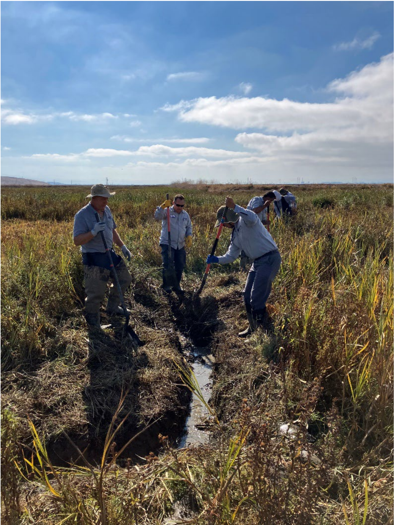
ACMAD ditch maintenance on Mowry Slough, September 24 th , 2024
